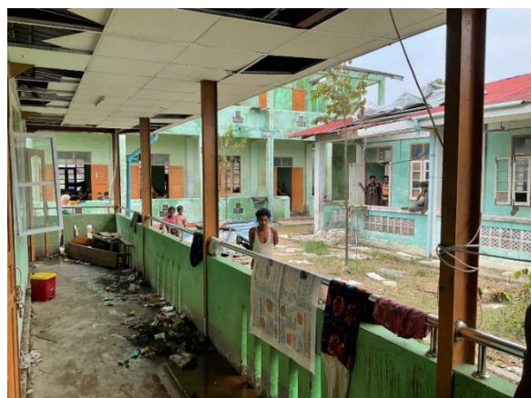
Thet Kae Pyin High School was used as shelter for 200-300 people. Sittwe, Rakhine. Credit: OCHA
