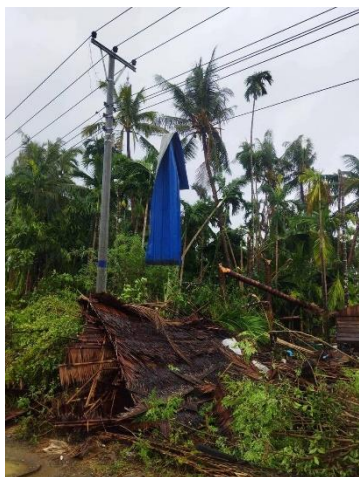
Destroyed house in Gwa township. Source: Twitter
