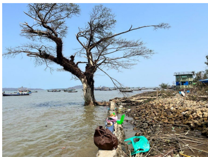
A jetty damaged by cyclone Mocha in Sin Tet Maw village. Pauktaw, Rakhine. Credit: OCHA
